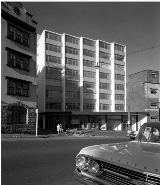
Figure 1 Home Units, 40 Bayswater Road, 1961, designed by HP Oser Fombertaux & Assoc Architects,. Photo by Max Dupain & Associates. (Source: State Library of NSW)
